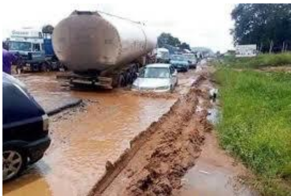
Figure 4. Damaged vehicles of commuters, stuck in mud for days because of the bad roads along Calabar Itu.
