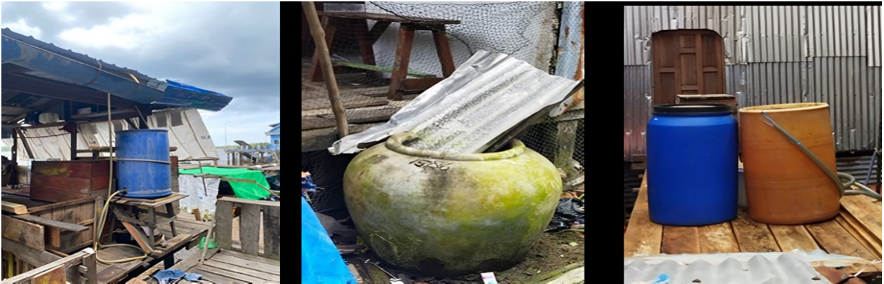
Figure 7. Condition of RWH buildings on a Household/Existing scale in Coastal Area Communities in Tanah Merah Village, Riau Province.
