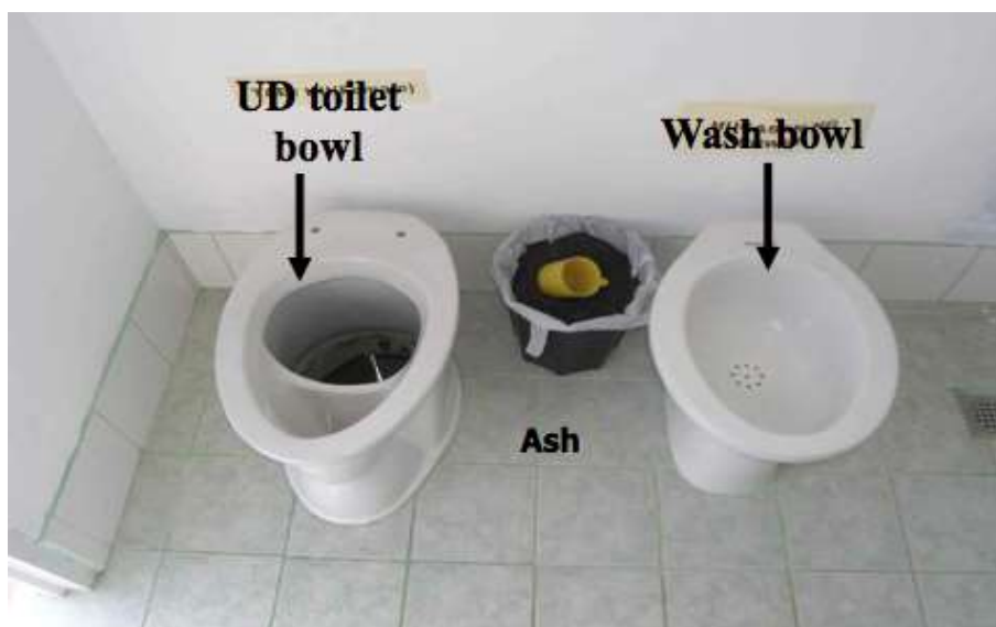
Figure 2. Urine diversion bowl toilets with separate wash bowl. Courtesy of the center for advance Philippine studies.
