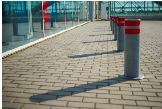
Figure 11. Anti-crash Bollard's system.
