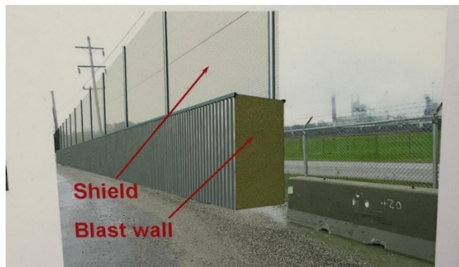
Figure 13. Steel plate with RC wall.
