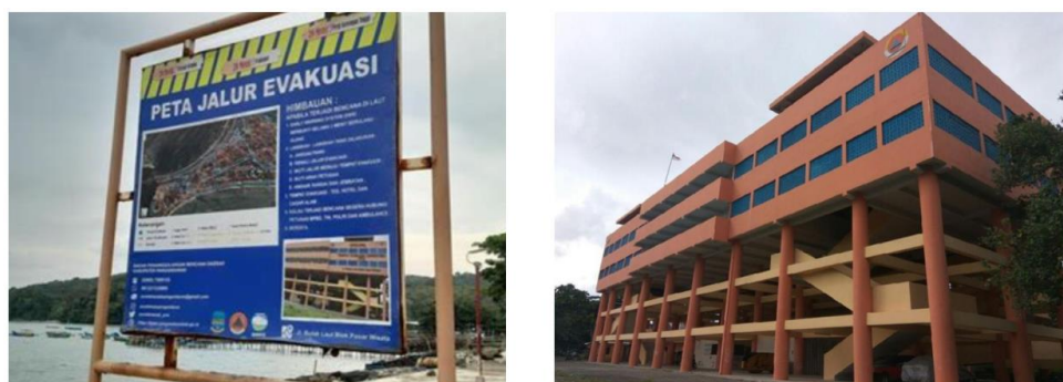
Figure 1. Evacuation routes and temporary shelter building (photo by authors).
