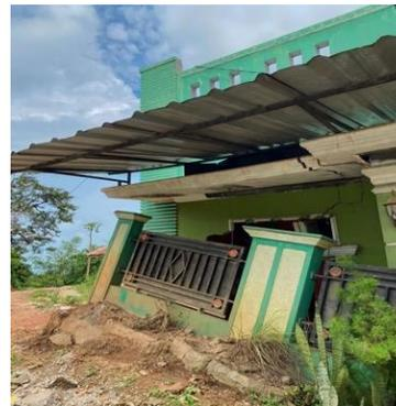
**Figure 1.** House damage due to ground movements caused by the Baribis Fault in Purwakarta, 2021.
