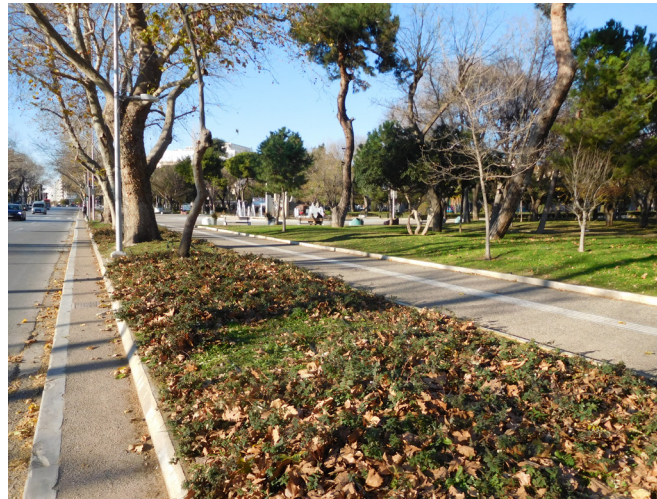
Figure 1. Upgraded local street for revitalization of urban area
