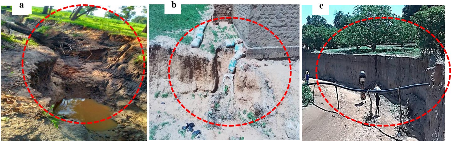
Figure 9. Erosion damage overview.
