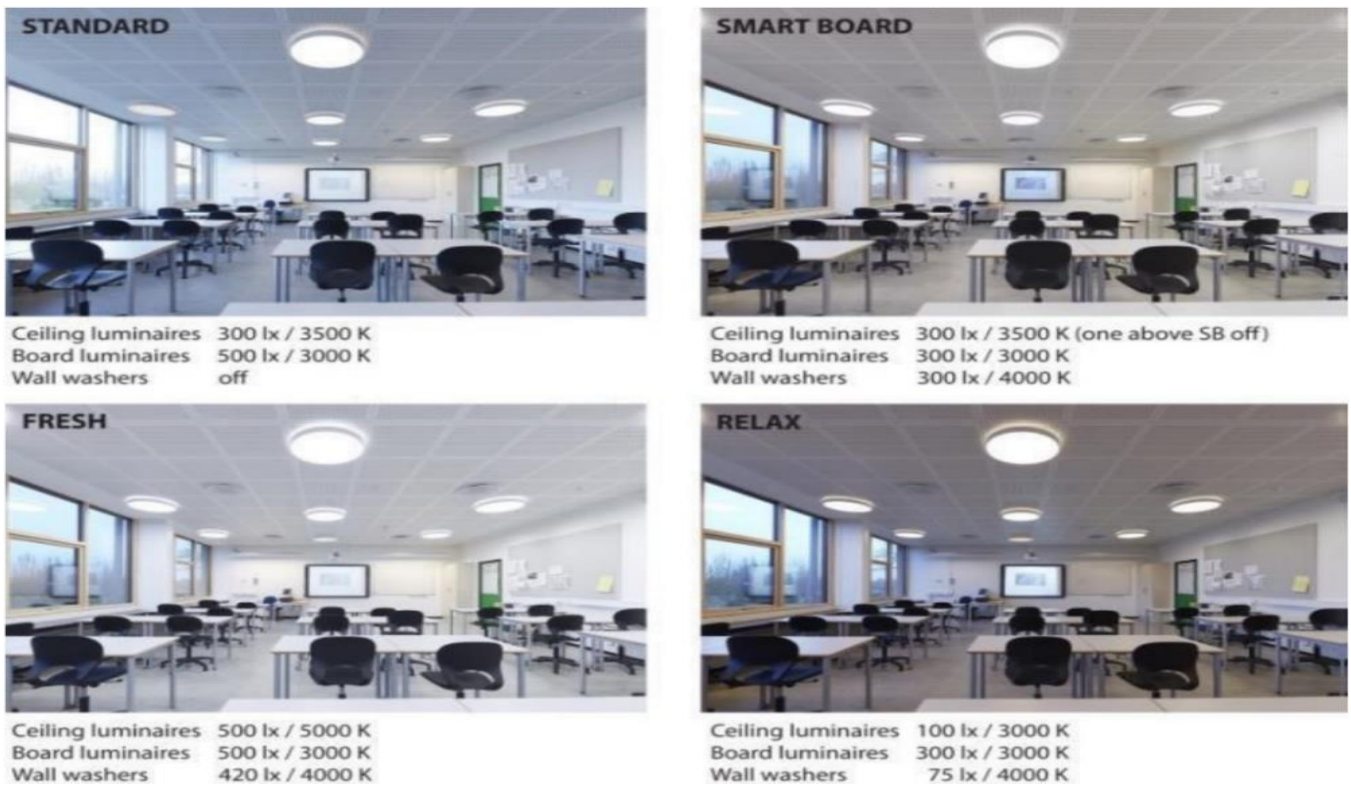
Figure 2. The illumination level and correlated color temperatures of different luminary groups were used in the four lighting scenarios (Lekan-Kehinde and Asojo, 2021).
