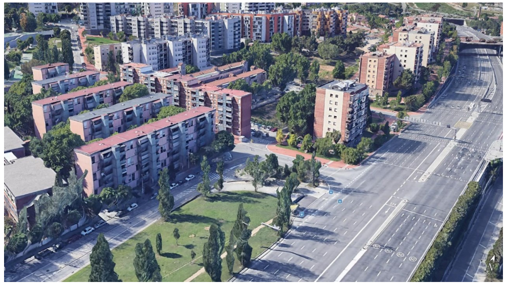
Figure 34. A similar perspective of Trinidad in 2020. Some of the privately constructed flats to the left have been demolished to make way for the new ring road. Some of the former public sector INV apartment blocks remain alongside the ring road. Photo: Google Earth.
