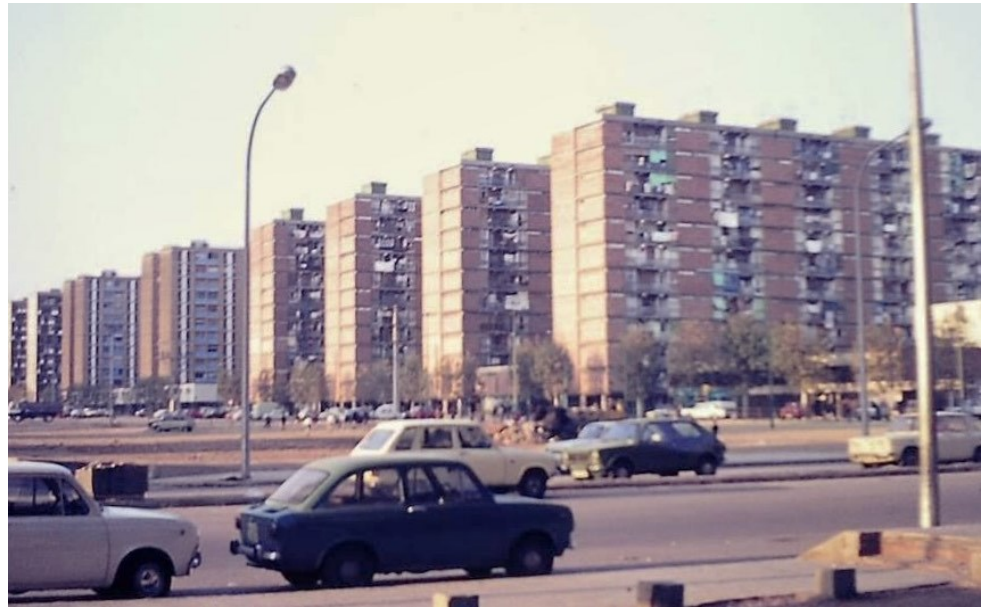
Figure 13. Sud-Oeste Besós in 1976. Some of the first large apartment blocks in the city displaying rationalist architecture. Photo: M. Wynn.
