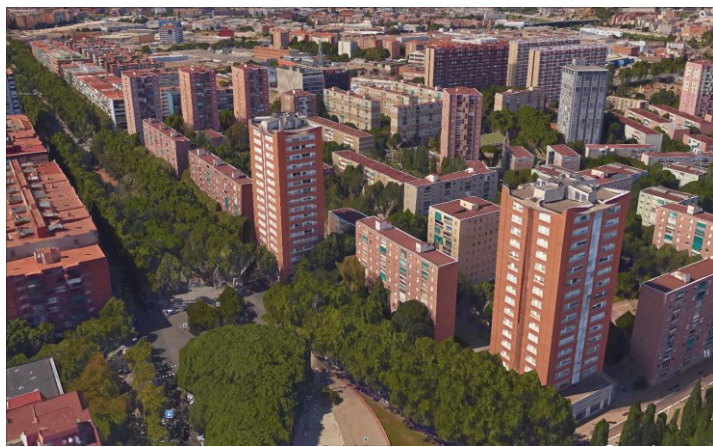
Figure 36. The La Paz estate in 2015. Compare with Figure 20 —green spaces, including the Rambla Prim, have been added around the tower blocks to improve the urban environment.
