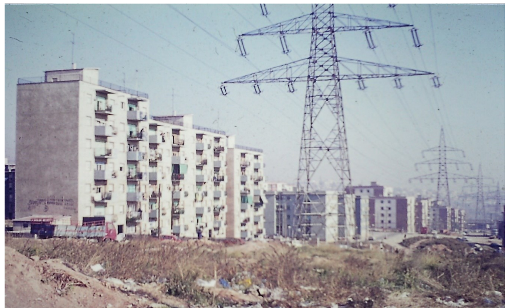
Figure 33. Part of the Trinidad neighbourhood in 1976—a mix of privately constructed apartment blocks to the immediate left and the public estates of the PMV and INV in the distance. Photo: M. Wynn.
