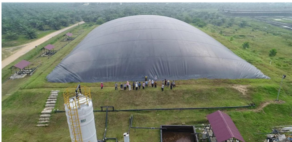
Figure 10. The government continues to encourage the development of renewable energy to be utilized massively by developing the potential for palm oil effluent or POME as a raw material for biogas which can be used as fuel for power plants.
