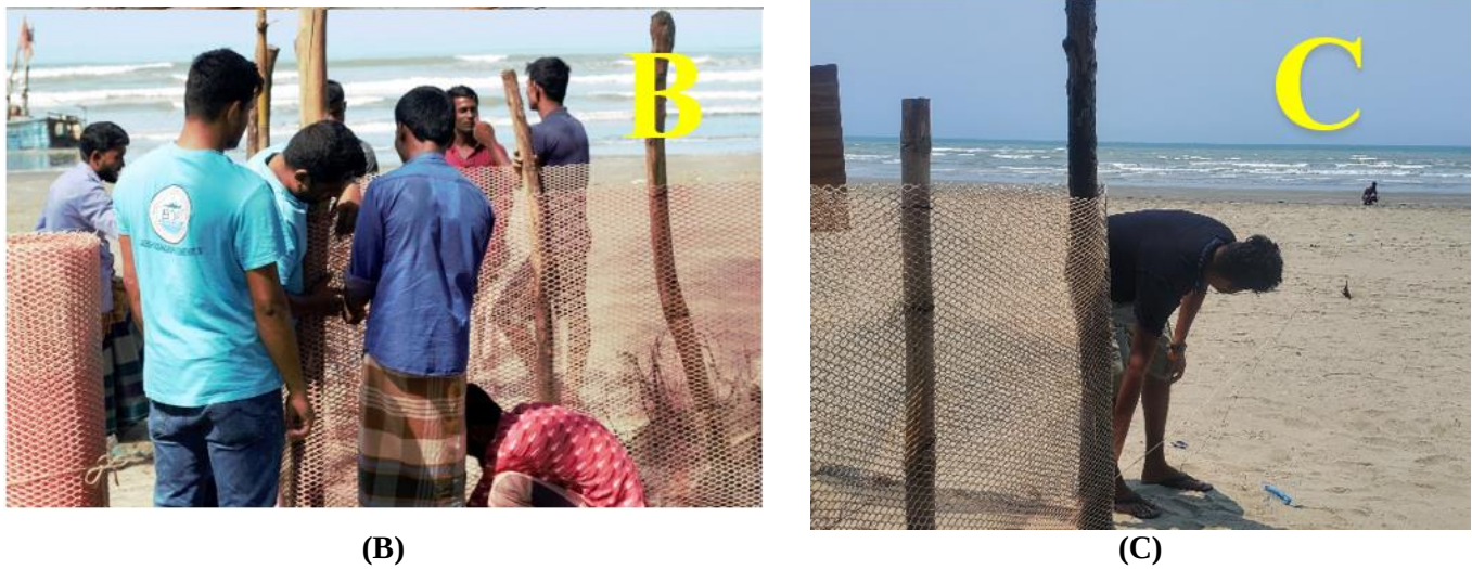
Figure 2. (A) construction of hatchery; (B) construction of hatchery; (C) measuring distance between high tide line and hatchery.
