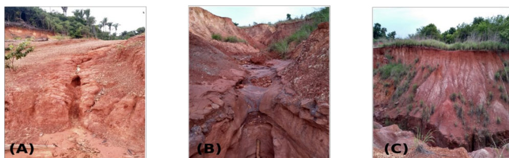
Figure 7. Erosive features found in the study area: (A) rills located in the municipality of União; (B) gully located in the municipality of Miguel Alves; (C) rills located in the municipality of União.
