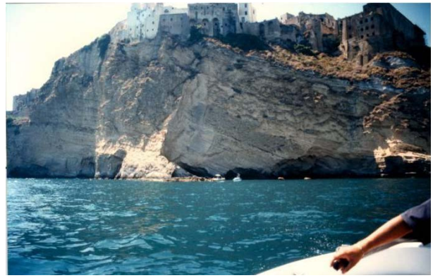
Figure 9. The Terra Murata coastal cliff towards the Corricella Bay, where the superimposition of two facies with different lithotechnical characteristics may be seen.
