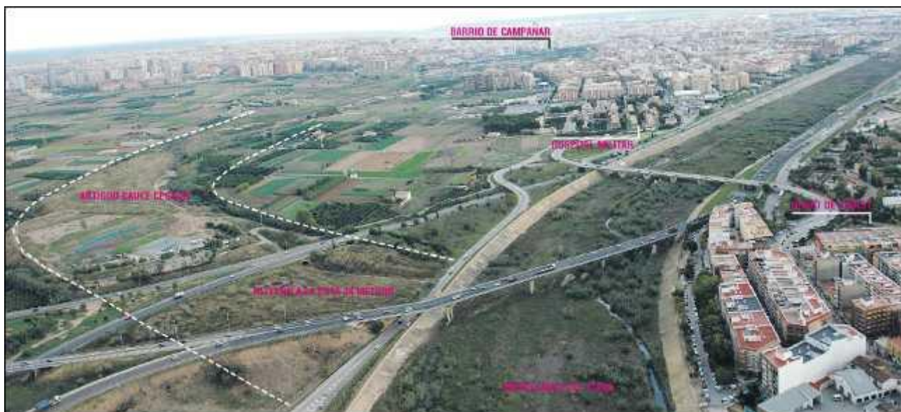
Figure 9. Aerial image showing the exact location where the river was diverted following the implementation of the Plan Sur.
