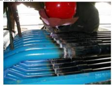
the welding port specifications  $\Phi 44.5$  (mm)  $\times 7.5$  (mm), the material is SA213 T91. Picture 1 pipe row welds
